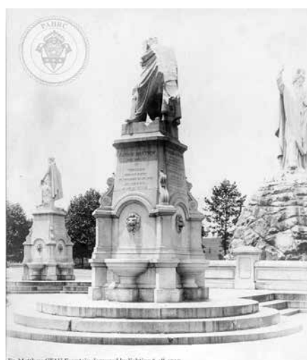
Fr. Theobald Mathew CTAU Fountain damaged by lightning, 6-18-1910.
